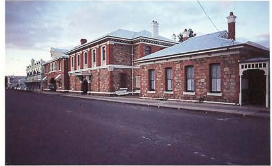
Public buildings, York, Western Australia. The post office, courthouse and police station were built in the 1890s and are registered with the National Estate. Photograph by Colin Beard.
